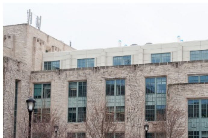
F-wing 4th floor, January 2012
