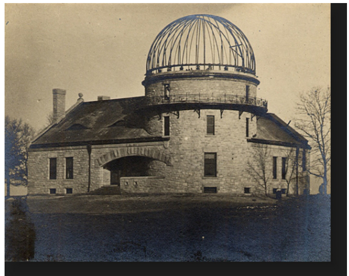
Early construction of the Dearborn Observatory dome, which was completed in 1875.
