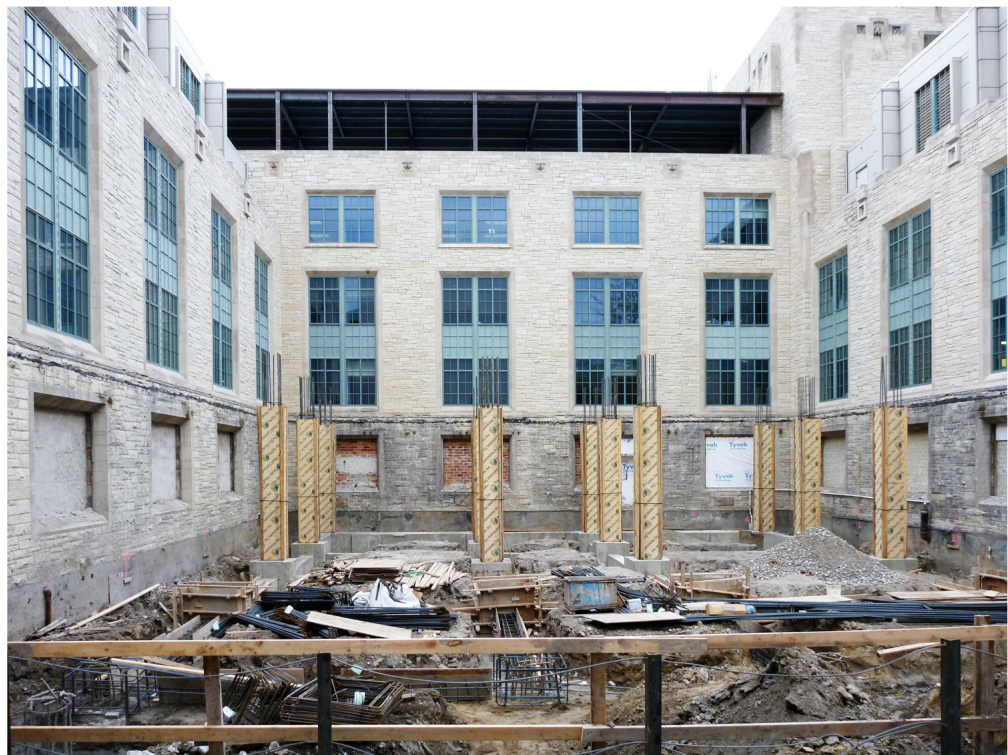
Concrete pillars of the new addition rise from the ground.
