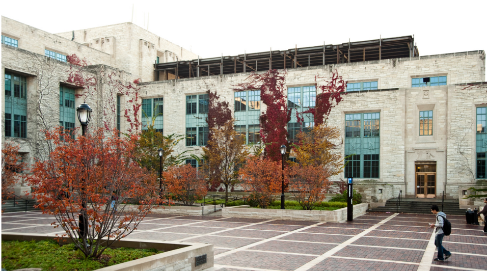
The beams outlining the frame of the new fourth floor of the F-Wing are almost in place.
